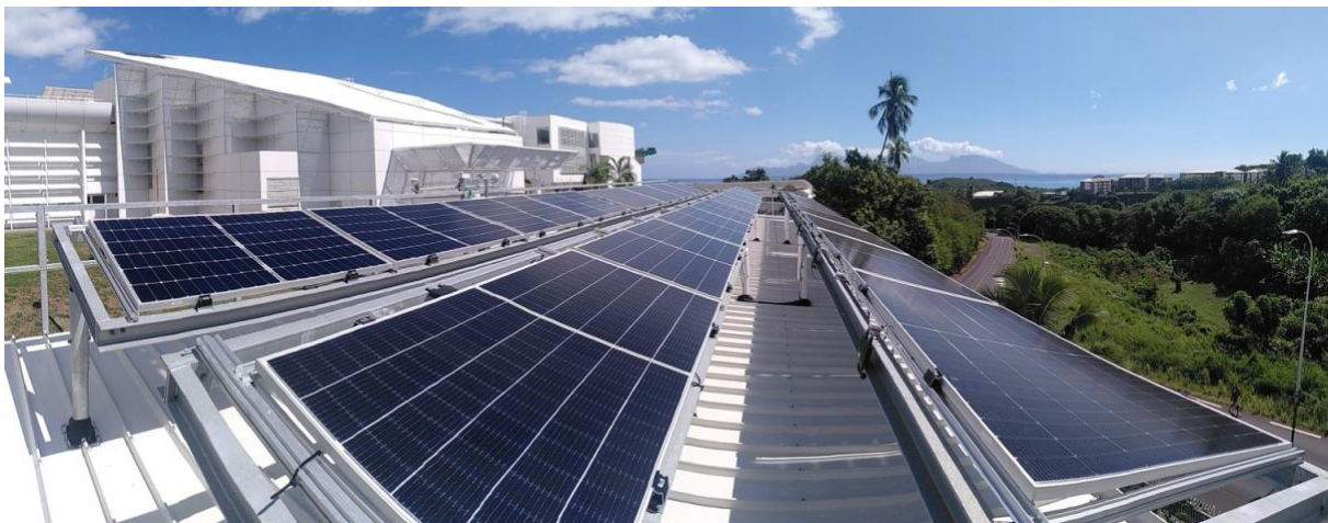
Figure 3 View of PVCAM platform (looking westwards)
