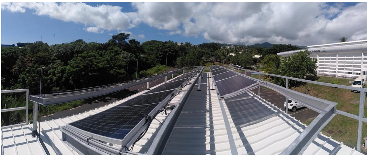
Figure 9 View of PVCAM (looking towards the East)
