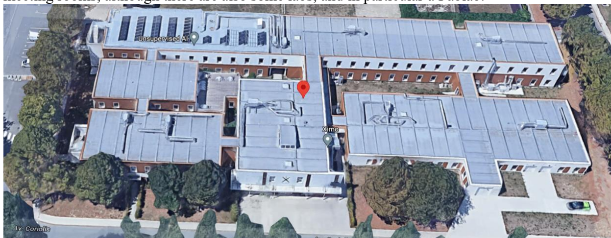
Figure 1 View of the Drahi-X Novation Center building (source: Google Maps)
