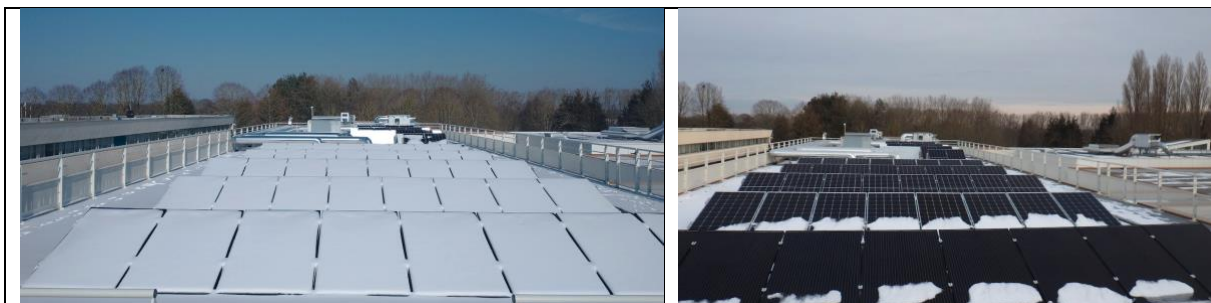
Figure 26 Snow on the installation on 10 Feb 2021 (left) and the state of the panels with still some snow for the ones 20°-tilted on 12 Feb (right).
